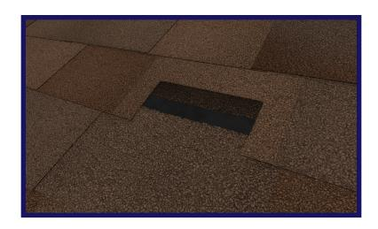
Locate and mark the location to which the base plate is to be attached. Cut the up-slope shingle the minimal amount needed to install base plate. This will ensure the flashing does not overhang the course below, protect the sides of the base plate, and ensure the best watertight protection for your installation.
