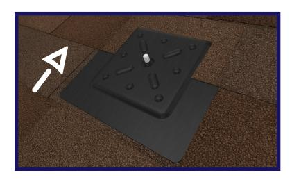
Slide the flashing over the base plate and through the stud. The flashing should be placed under the course of shingles that was cut in Step #1. The down-slope edge of the flashing should be approximately even with the bottom of the shingle. The flashing should not overhang the down-slope shingle more than 1".
