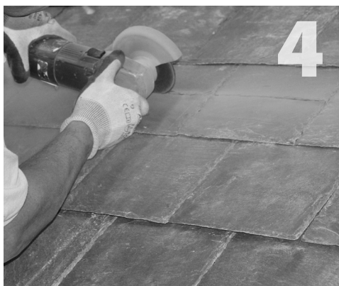
Using a cutoff wheel in a grinder, score the slate above the mounting area at 4 inches above the center of the QB-1 location. In step 5, you will remove the slate below the score line, which will allow you to slide the flashing up under the remaining slate in step 10.
