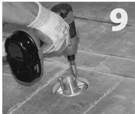
Prior to mounting to the roof, seat the grade-8 cap screw (item 1) through bottom of QB-1. Secure the QB-1 to the rafter with (2) 5/16" lag screws (item 3) and tighten to a snug fit.
