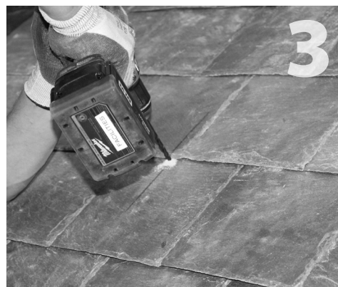
Using a masonry drill bit, drill a pilot hole at the center of the QB-1 location you marked in step 2. This drill bit should match the size of the guide bit
