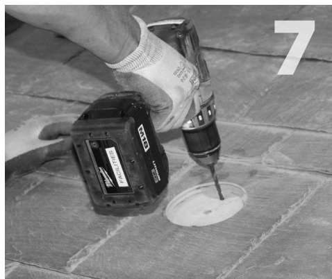
Using QB-1 (item 2) as a guide, align two clearance holes vertically with the center of the rafter. Mark the center of these 2 holes. Drill 7/32" pilot hole at each of the 2 marks. Hold drill square to rafter. Do not use QB-1 as a drill guide.
