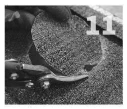
Mark a circle and cut out with aviation tin snips. The hole should be large enough to leave about a <sup>1</sup>/<sub>2</sub>" gap between the cone flashing and the panel. See Getting Started: Cutting Steel Shingles.
