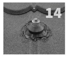
Slip the EPDM rubber collar over the post and slide collar down to the flashing.
