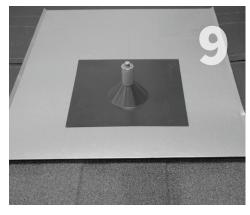
Slide the flashing over the post/standoff.
