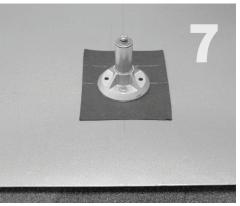
Screw the post into the grade-8 cap screw in the QB-1 mount. Use a pair of channel lock pliers to tighten it down.
