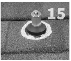
Slip the EPDM rubber collar over the post and slide collar down to the flashing.
