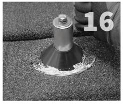
Cover sealant with shingle manufacturer's color matched stone granules. **See Getting Started: Applying Granules.** Install the L-foot using the hardware supplied as required.
