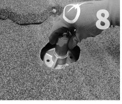
Screw the post onto the grade-8 cap screw in the QB-1 mount. Use a pair of channel locks to tighten it down.
