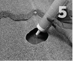
Add sealant compatible with contacted materials and environmental conditions to the pilot holes.
