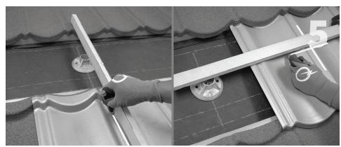
Mark off the location of the center of the mount on the underpan made specifically for your roofing type.
