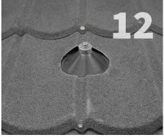
Reinstall the panel over the flashed QB-1 mount and post using the screws removed in step 1.
