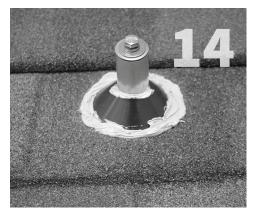
Apply a heavy bead of sealant to the area between the shingle panel and the flashing. Smooth sealant *without removing large amount of sealant*. Sealant should maintain thickness as much as possible. Apply a bead of sealant where the post meets the flashing.
