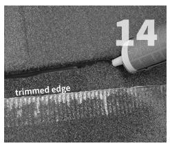
**Interlocking type shingles** may require trimming off the interlock of the secondary 1/2 length panel. **(See Getting Started)** Apply sealant where the panels interlock, then place the ½ length panel over the flashing and slide the trimmed edge up under the panel above. Apply a second bead of sealant where this edge is embedded.
