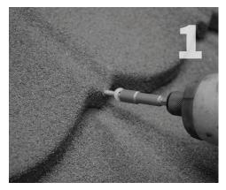
Remove screws from metal shingle panel and remove the panel at the mount location.
