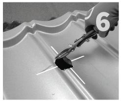
Mark a circle and cut out with aviation tin snips. The hole should be large enough to leave about a  $\frac{1}{2}$ " gap between the underpan and the QB-1 mount.
