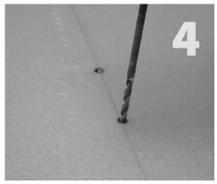
Drill pilot holes through the clearance holes and into the rafter using a  $7/_{32}$ " bit. Add sealant compatible with contacted materials and environmental conditions.
