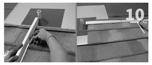
Mark off the location of the center of the mount and the flashing cone on the shingle panel that was removed in step 2.
