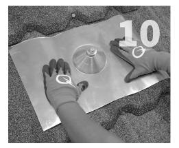
Mold the dead soft aluminum flashing cone to fit the contours of roofing panel.
