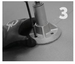
Mark the location for your mount over the center of the rafter and drill (2) <sup>3</sup>/<sub>8</sub>" clearance holes through the underpan. See: **Getting Started** for working with gaps beneath the underpan.
