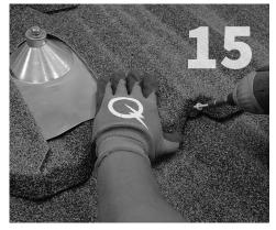
Screw all roofing panels down.
