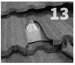
**For non-interlocking type shingles**, insert the cut ½ length panel over the flashing and under the panel above.
