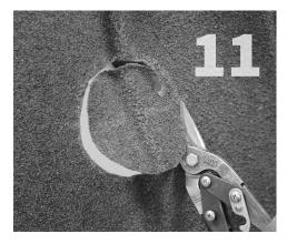
Mark a circle and cut out with aviation tin snips. The hole should be large enough to leave about a 1/2" gap between the cone flashing and the panel. See Getting Started: Cutting Steel Shingles.
