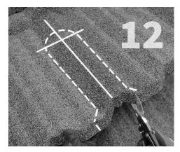
Cut an opening around the cone flashing and down to the bottom of the  $\frac{1}{2}$  length panel.
