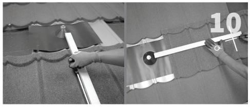
Mark off the location of the center of the mount and the flashing cone on the panel that was removed in step 2.
