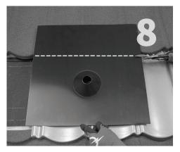
Trim the cone flashing as required to fit the underpan.
