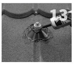
Apply a heavy bead of sealant to the area between the panel and the flashing. Smooth sealant without removing a large amount of sealant. Sealant should maintain thickness as much as possible. Apply a bead of sealant where the post meets the flashing.
