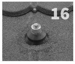
Apply color matched stone granules to the sealant. Install the L-foot using the hardware supplied as required.
