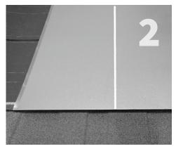
Install the manufacturer's interlocking underpan made specifically for your roofing style. Mark off rafter on the underpan.
