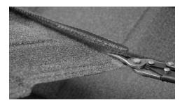
When using the sandwich method of flashing on interlocking type shingles, it may be necessary to remove the interlock edge on the secondary (top) layer of shingles. Bend up the interlock, then cut it off at the bend using a pair of tin snips.
