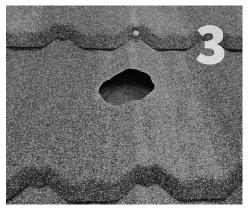
Remove the shingle course and cut a 4" hole in the roofing panel using tin snips. See Getting Started: Cutting Steel Shingles.
