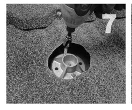
Bolt the QB-1 mount to the rafter using (2)  $5\!\!/_{16}$  lag bolts, and tighten to a snug fit.
