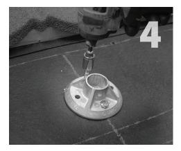
Fill pilot holes with sealant compatible with contacted materials and environmental conditions. Bolt the QB-1 mount to the rafter with (2) %6" lag bolts and tighten to a snug fit.
