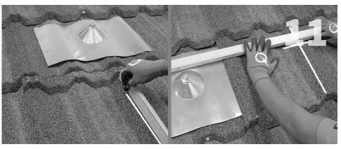
Mark off the location of the center of the mount and flashing cone on a secondary ½ length panel of the same roofing. Contact the shingle manufacturer to source additional panels to match your roof type.
