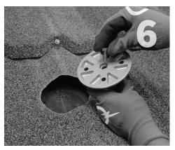
Insert grade-8 cap screw into the bottom of the QB-1 mount.
