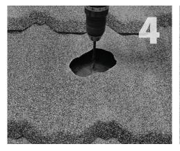
Drill (2) 7/32" pilot holes into the center of the rafter.
