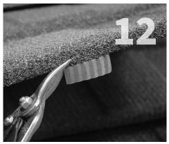
Use tin snips to cut (2) 2" notches in the bottom interlocking edge of the next panel. The notches should be centered approximately 4" apart, centered below mount. Granules may be added for aesthetic purposes. See Getting Started: Applying Granules.
