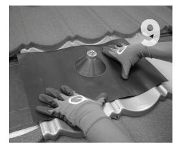
Mold the dead soft aluminum flashing cone to fit the contours of the underpan.
