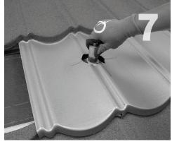
Lay the underpan into place. Screw the post into the grade 8 cap screw in the QB-1 mount. Use a pair of channel lock pliers to tighten it down.
