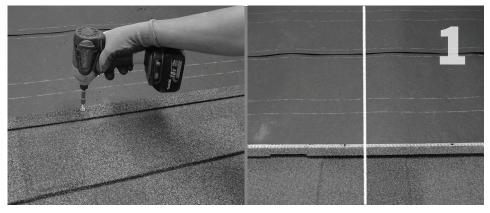
Remove the panels at the mount location to the course below your lowest mount. For new construction, install roofing panels up to the course below your lowest mount. Locate the rafter on the roof.
