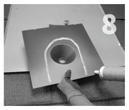
Apply an upside down "U" shape of sealant to bottom of the cone flashing.
