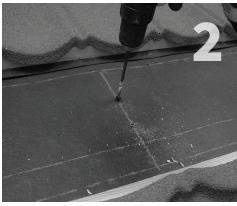
Mark the center of the rafter, layout the mount within the shingle coursing, drill (2)  $7/_{32}$ " pilot holes into the center of the rafter.
