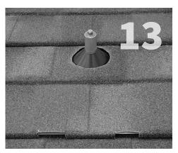
Reinstall the shingle panel over the flashed QB-1 mount and post using the screws removed in step 1.
