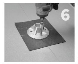
Cut an approximately  $5" \times 5"$  square of roofing felt. Bolt the QB-1 mount to the rafter on top of the square of felt using (2)  $\%_{16}"$  lag bolts, and tighten to a snug fit.
