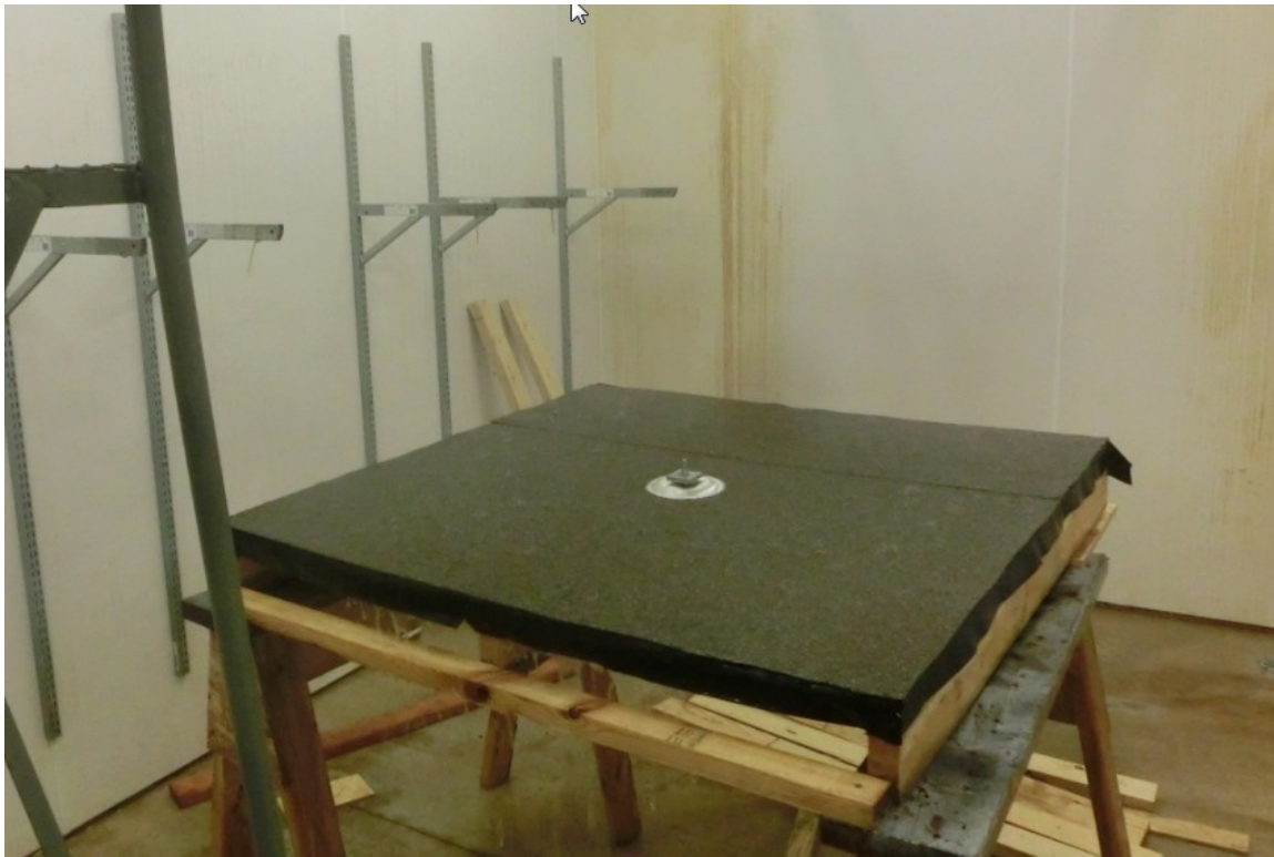
Photo 5: Test Deck Sample at 1/4:12 Pitch
