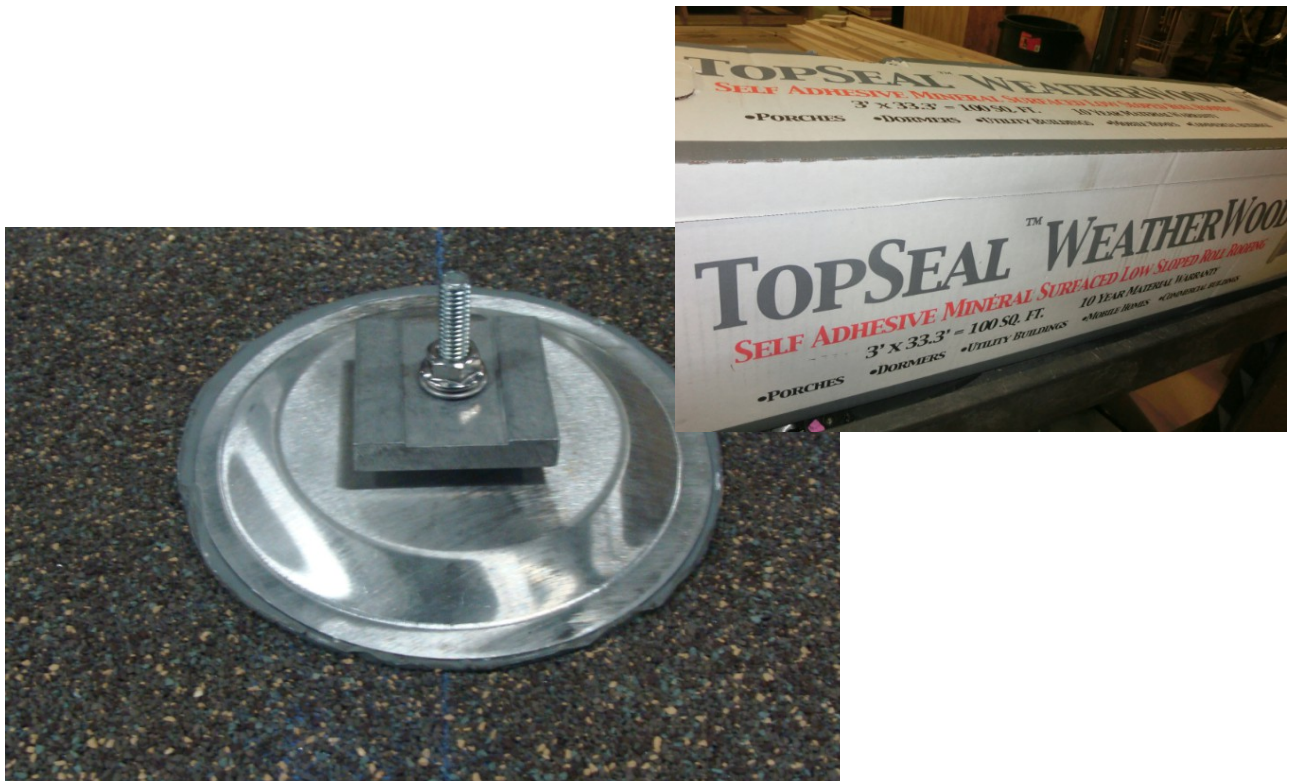
Photo 2: SimpleGrip Assembly Installed
