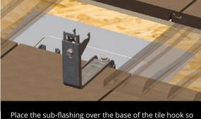
Place the sub-flashing over the base of the tile hook so the flashing covers the entire base.
