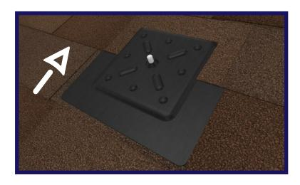
Slide the flashing over the base plate and through the stud. The flashing should be placed under the course of shingles that was cut in Step #1. The down-slope edge of the flashing should be approximately even with the bottom of the shingle. The flashing should not overhang the down-slope shingle more than 1".
