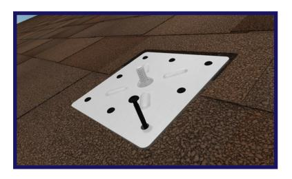
Attach the base plate to the roof. All fastener holes should be used. Fasteners securing to the roof sheathing should be a minimum of 2" long.
