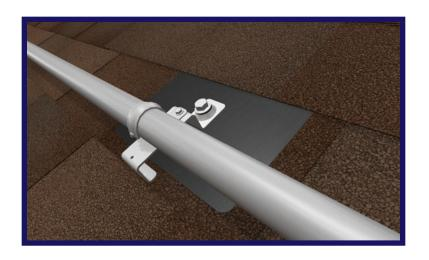
Drive the lag bolt down into the roof deck using an impact driver. The visual indicator for proper torque is when the EPDM on the underside of the bonded washer begins to push out the sides as the washer compresses. Do not over torque.
