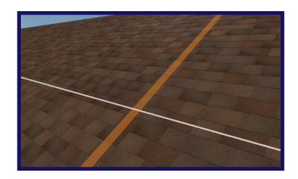
Snap horizontal lines across the roof to mark the mount rows, then locate the rafter and mark the installation position of each GF-1 flashing.
