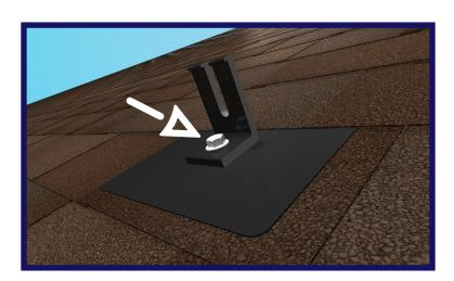
Drive the lag bolt down into the rafter using an impact driver.
