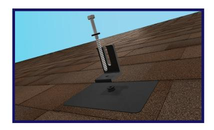
Thread the EPDM bonded washer onto the lag bolt followed by one of EcoFasten's compression brackets and then insert the lag bolt into the gasketed hole in the flashing.
