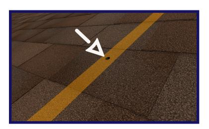
Drill a 7/32" pilot hole into the rafter or structural member for the lag screw. Backfill with sealant compatible with the roof type.
