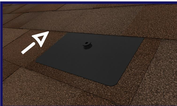
Slide flashing up under the next row of shingles directly above the pilot hole, taking care to align the hole in the flashing with the pilot hole.
