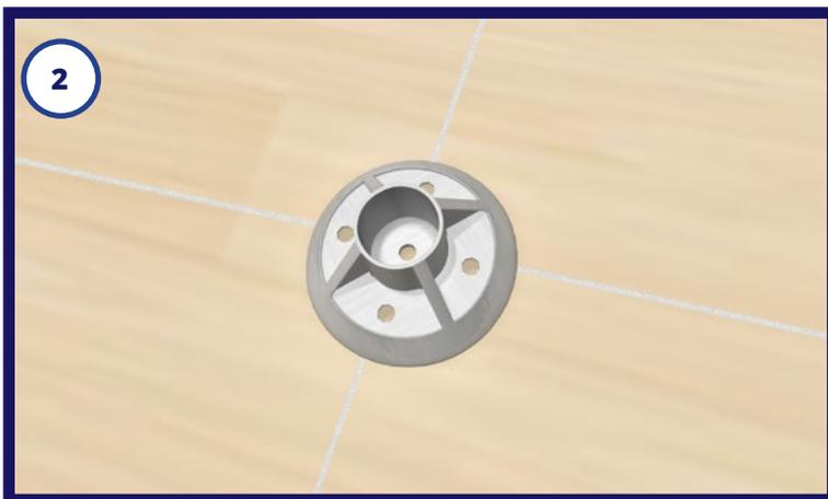
2. Align QB-1 Base vertical holes over center rafter mark and horizontal holes over the snapped row line. Mark holes for drilling. Remove QB-1 Base and drill two 7/32" pilot holes into the rafter. To mount directly to the deck, follow the recommendations of the engineer of record.
