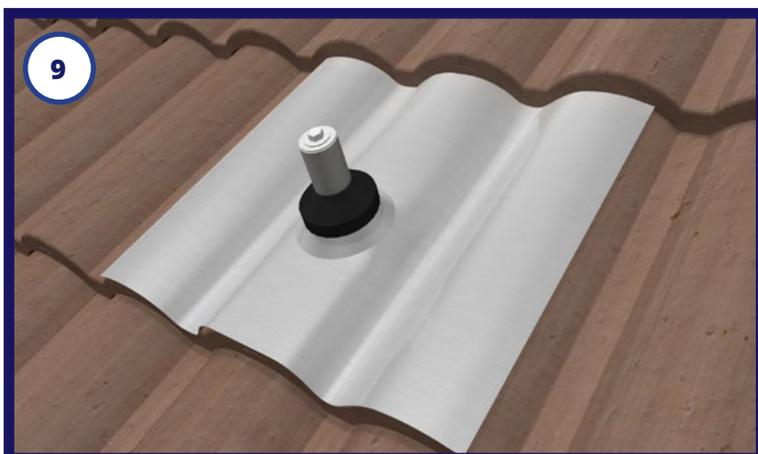
9. Install the tile-level flashing. It is possible to use the 18 x 18" flashing or other third party cone flashing. EcoFasten's 18 x 18" flashing is malleable, so it is possible to shape the flashing to conform to the shape of the tiles.
