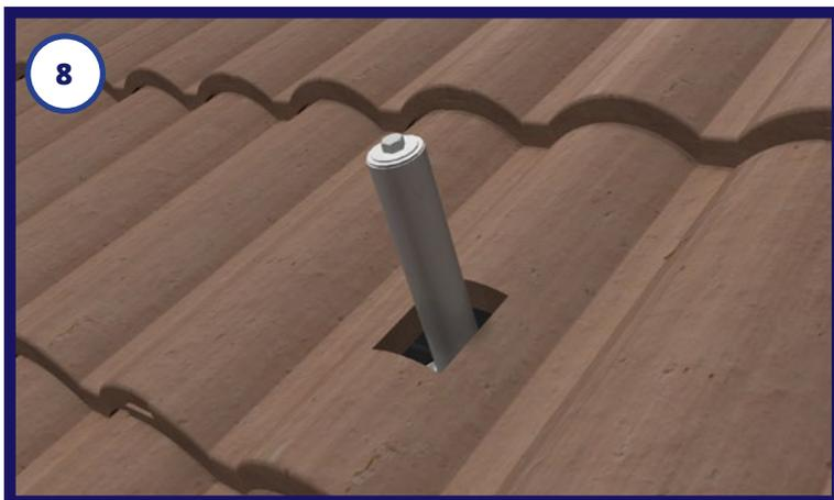
8. Install tile and cut to allow post to pass through. Place cut tile back in position.
