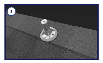
5. Install shingles on the roof up to the point that the shingles reaches the installed mount. Cut a hole or half circle in the shingle course around the QB-1 Base.
