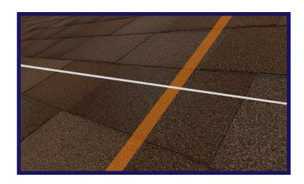
Snap horizontal chalk lines to mark the position of each row. Find the rafters and mark the position for installation.
