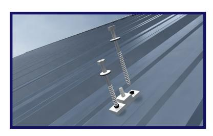
Thread the 5/16" EPDM bonded sealing washers onto the 5/16" lag bolts and insert the bolts into the top of SimpleSeal bushings.
