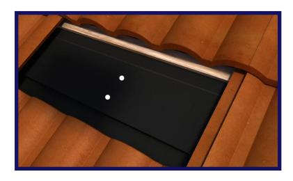
Drill two pilot holes using 1/8" bit to a depth of 2 3/4". Be sure lags go into center of rafter for strongest attachment. Pilot holes reduce rafter splitting. Fill pilot holes with appropriate sealant and align lag holes over the pilot holes.
