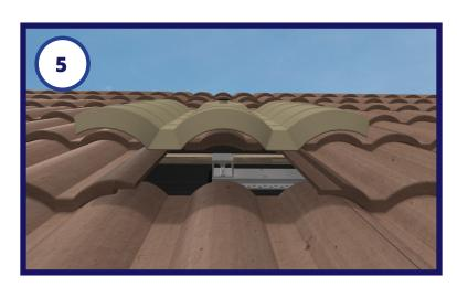
5. Install the flashing so that the hole in the flashing lines up with the selected hole in the base plate pedestal below. The top of the flashing should be positioned under the tile above.
