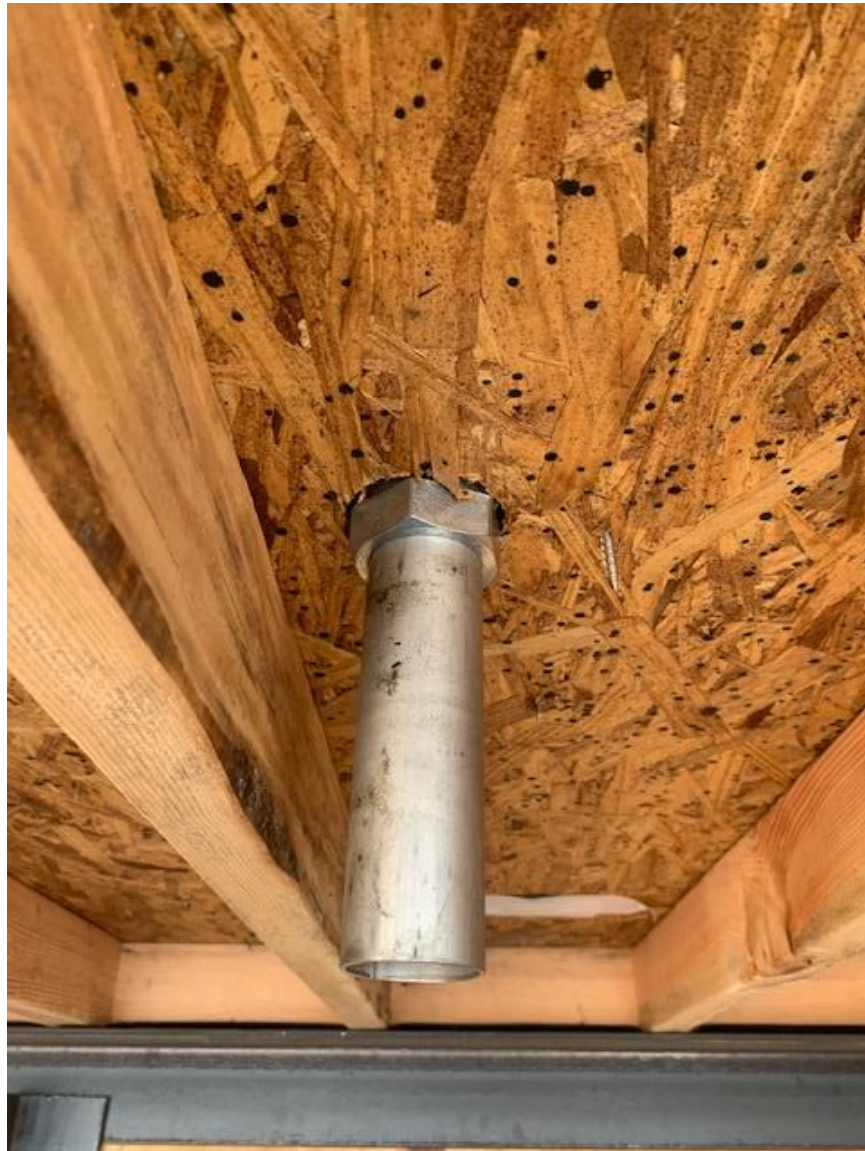
Photo No. 2 Underside of the Test Deck
