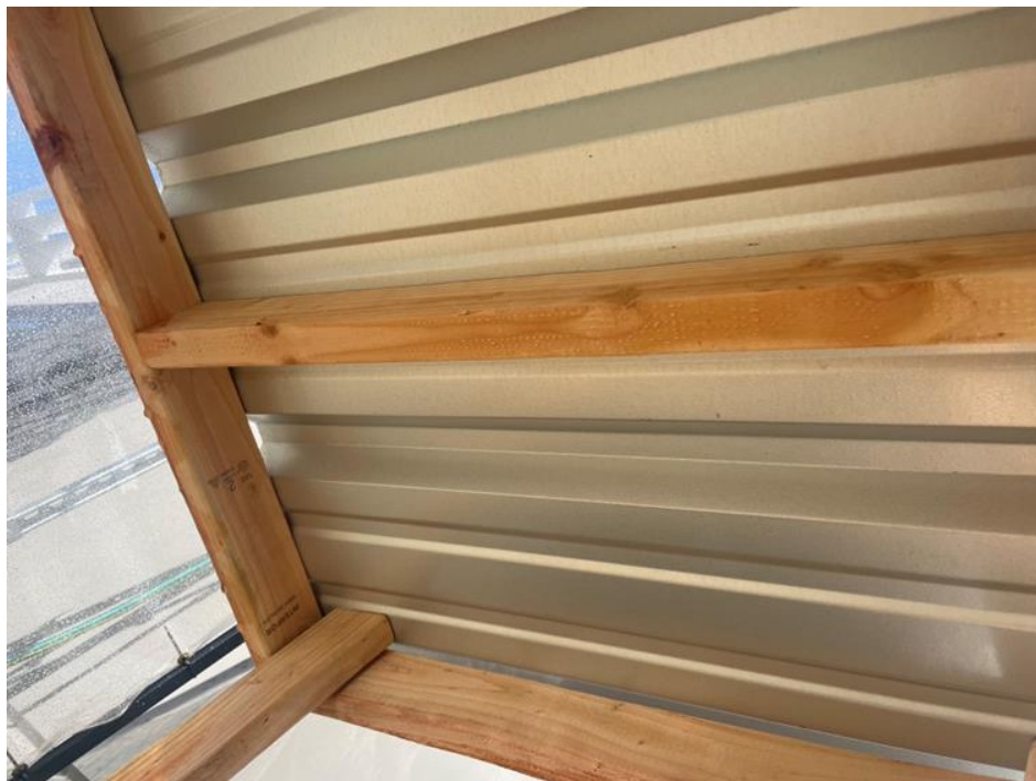
Photo No. 4 Underside of Test Desk After Test – no visible water penetration
